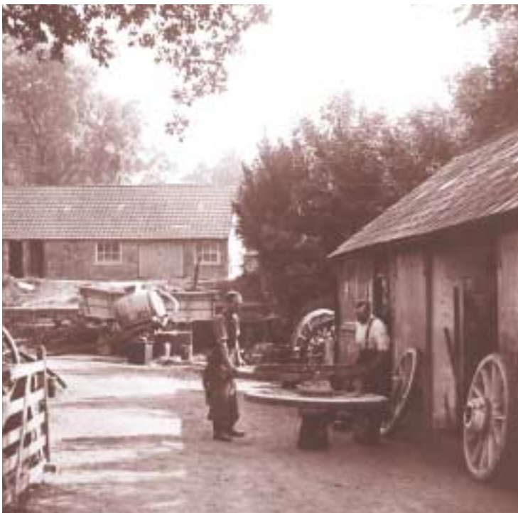
Tying wagon wheel with iron hoop. Maidstone Forge, Kent (1938)
