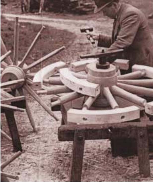
Hammering ash felloes onto spokes (1941)
