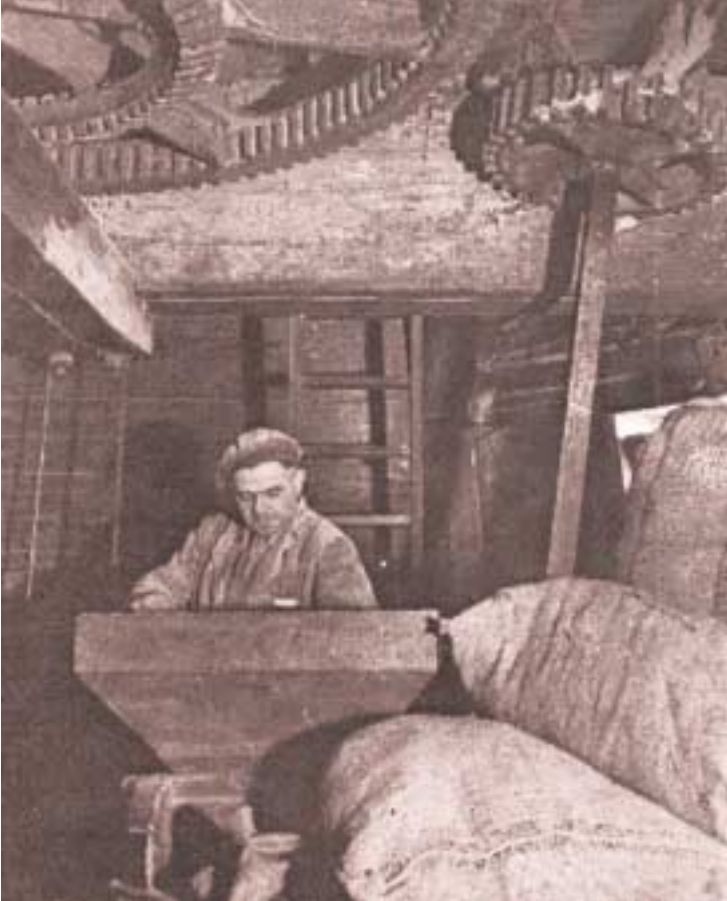
Union Mill, Cranbrook, Kent (1952)
